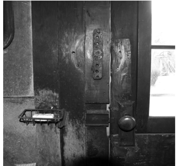
FIGURE 20. View of latching mechanisms at back door.
