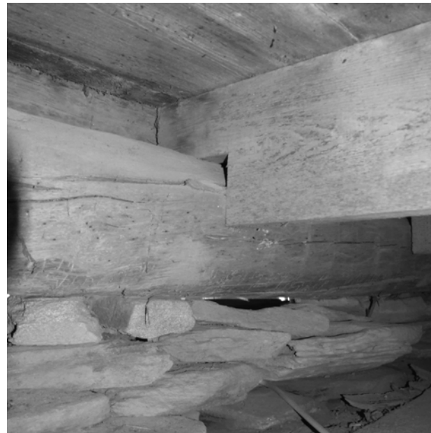
FIGURE 62. View of front sill of log pen near northwest corner with typical floor joist connection.
