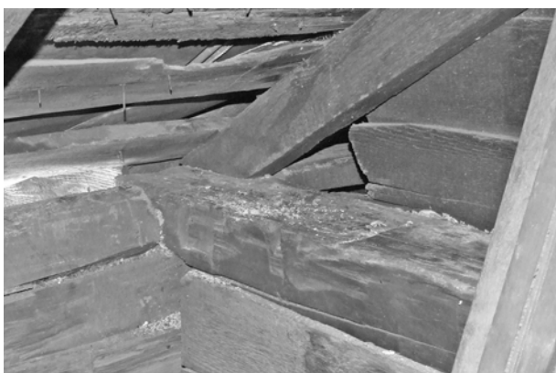
FIGURE 63. View of lap joint connecting top plates at southwest corner of log pen.
