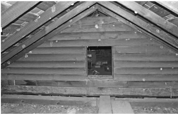
FIGURE 93. View east in attic of 1925 addition, showing original antebellum gable siding on log
