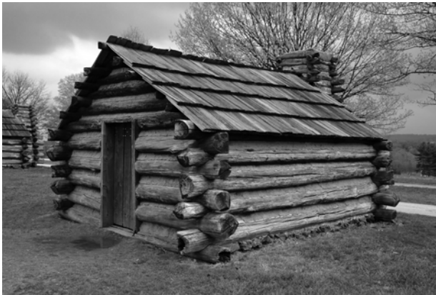
FIGURE 29. A replica of the crude log huts built with simple saddle notches and purlin roofs by Washington’s troops at Valley Forge. (Dan Smith, Wikipedia Commons)
