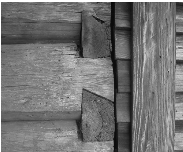
FIGURE 61. View of typical half-dovetail joinery in log walls.
