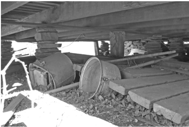
FIGURE 75. View northwest under 1927 addition, showing supports added at midpoint of floor joists.
