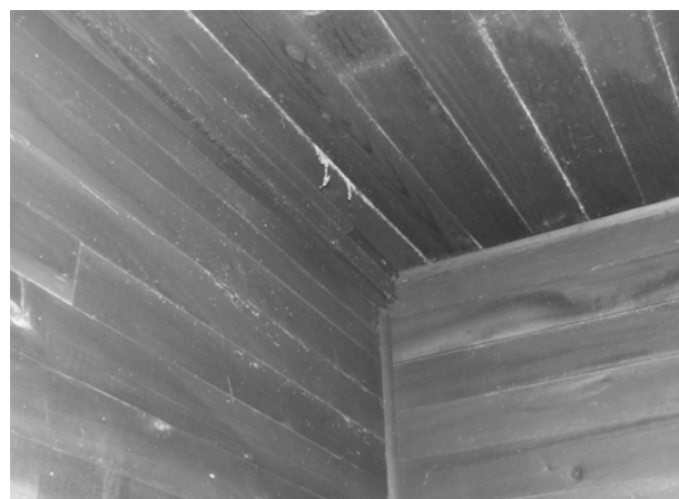
FIGURE 130. View of the junction of walls and ceiling at southwest corner of Room 103, showing typical quarter-round trim. The projecting ledger flanked by quarter round runs at the top of the wall on the left.
