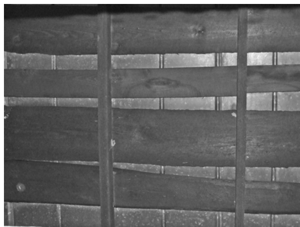
FIGURE 107. View of typical decking on roof of 1927 addition. Note absence of nails protruding through the decking suggesting that it was never covered with wood shingles.
