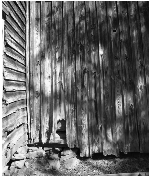
FIGURE 25. View of board-and-batten siding on rear of log pen.
