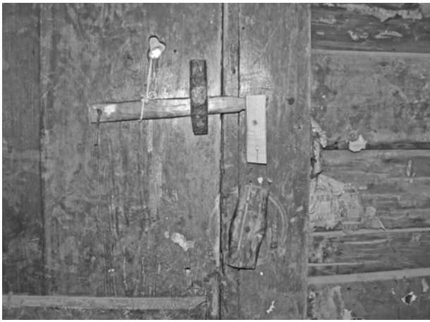
FIGURE 117. View of pivot latch and repaired string latch on original front door, Room 101.
