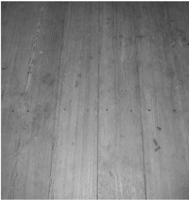
FIGURE 29. View of typical quarter-sawn pine flooring used in the log pen.
