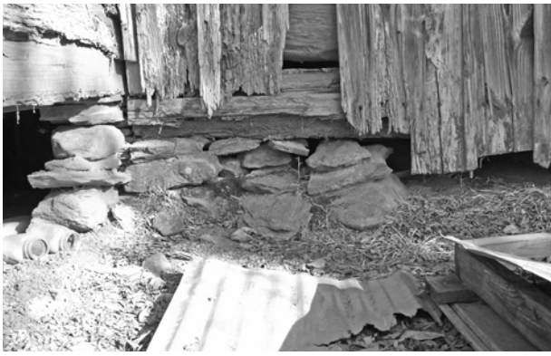
FIGURE 45. View of foundation piers and underpinning at junction of the rear of the log pen and the northeast corner of the 1927 addition.
