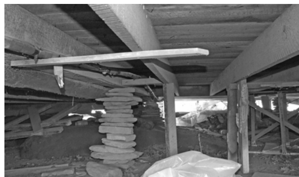
FIGURE 51. View south under 1925 addition showing stone pier near center of west sill of log pen. This pier was probably installed when the cellar entrance was removed for construction of the addition.
