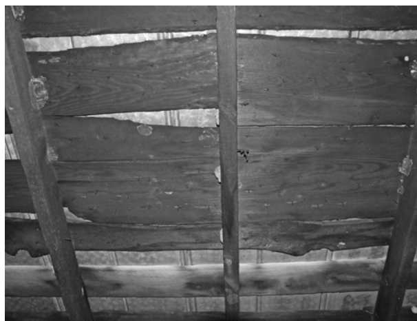
FIGURE 106. View of decking on south slope of log-pen roof, showing typical 1840s slab-wood decking.
