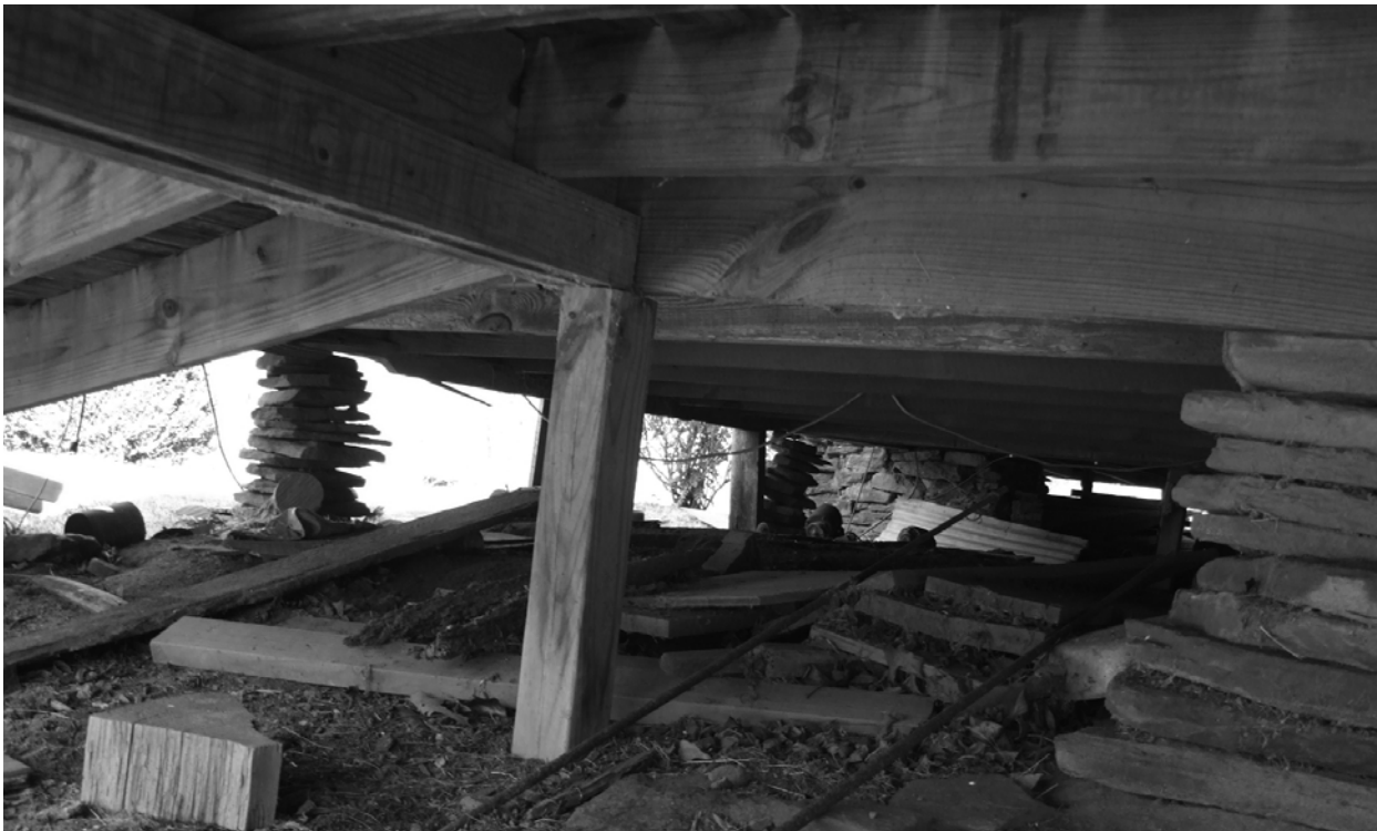
FIGURE 2. View of typical wooden post installed to reinforce the house's floor framing but which can provide entry to termites.
