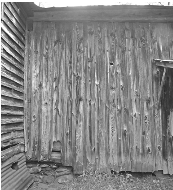
FIGURE 95. View of typical 1920s board-and-batten siding on rear of log pen.
