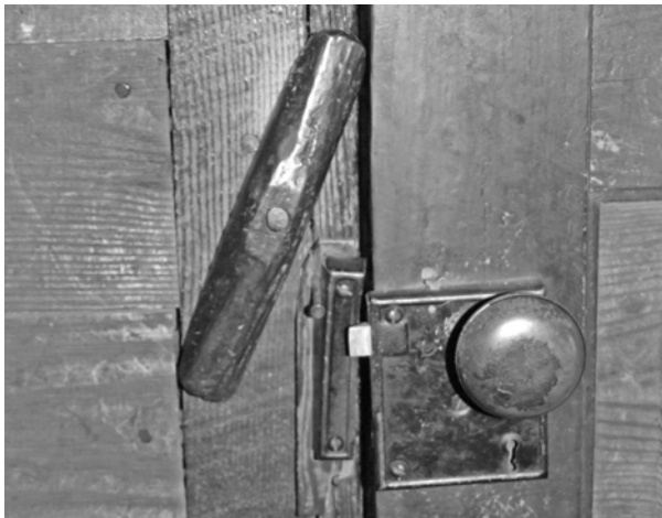
FIGURE 127. View of rim lock and pivot latch on door between Rooms 103 and 104.
