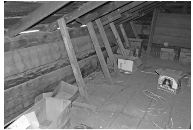
FIGURE 71. View of modern wooden braces installed at west end of rear (south) side of log pen.
