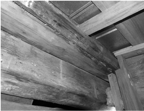
FIGURE 66. View of top of front (north) wall of log pen, showing projecting log that forms the top plate. The 2" by 4" ledger nailed to the front of the plate was probably part of the construction of the original front porch.
