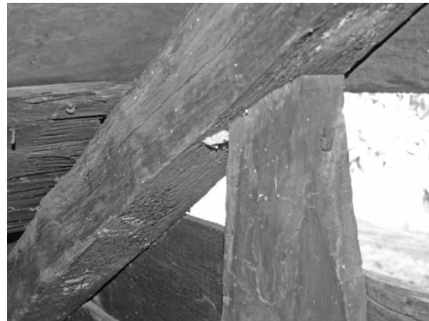
FIGURE 69. View of typical stud-rafter connection at east gable of log pen.
