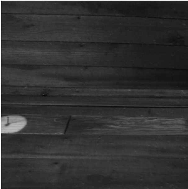
FIGURE 26. View of sooty walls in Room 103, with light circle at left where a circular-saw blade hung for many
