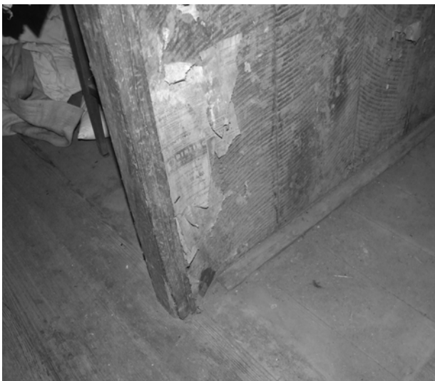
FIGURE 119. View of connection of curtain wall to floor, showing cleats that hold the wall in place.
