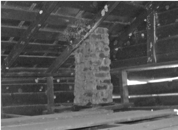
FIGURE 60. View of stove flue in attic of 1927 addition.
