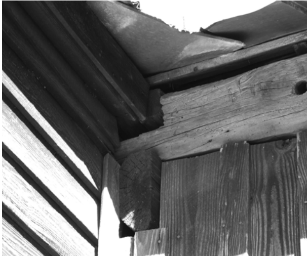
FIGURE 22. View of intersection of log pen and kitchen wing, illustrating the numerous openings in the exterior finishes.
