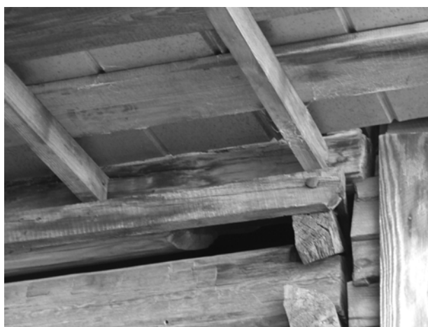
FIGURE 78. View of rafter connection for 1996 addition at front of log pen. southeast in attic of 1927 addition showing typical framing.
