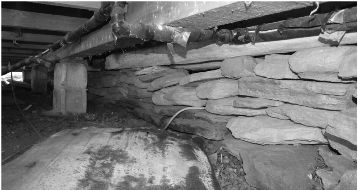
FIGURE 3. View of rock underpinning front sill of log pen.
