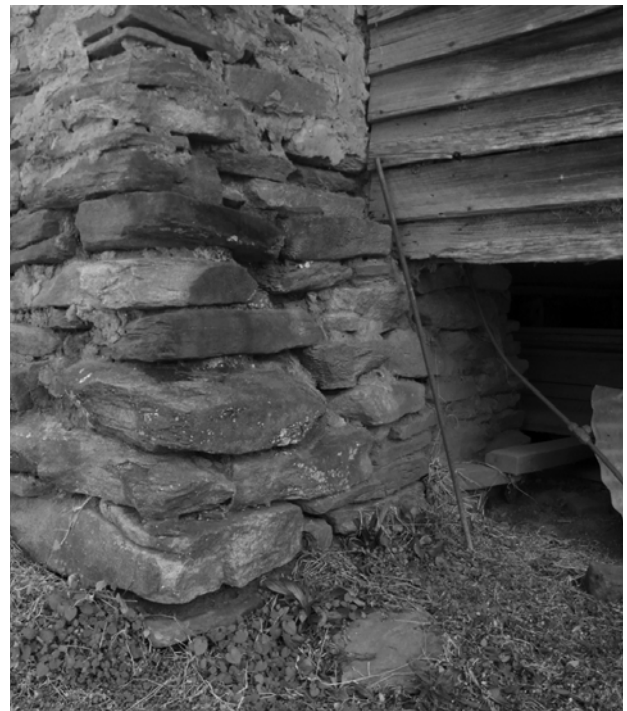
FIGURE 7. View of chimney and hearth base for fireplace in Room 103.
