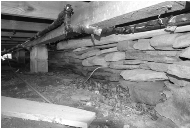
FIGURE 46. View east-southeast of stone underpinning under front sill of log pen.
