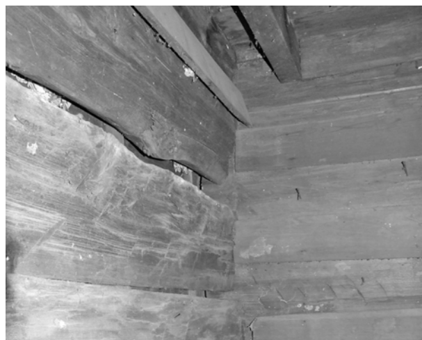
FIGURE 114. View of northwest corner of log pen, illustrating significant gaps that exist between some logs.
