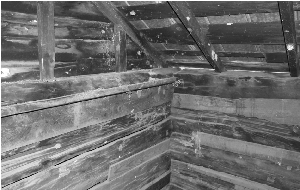
FIGURE 11. View of southeast corner of log pen. All of the material visible here, except the metal roofing, dates to the 1840s.
