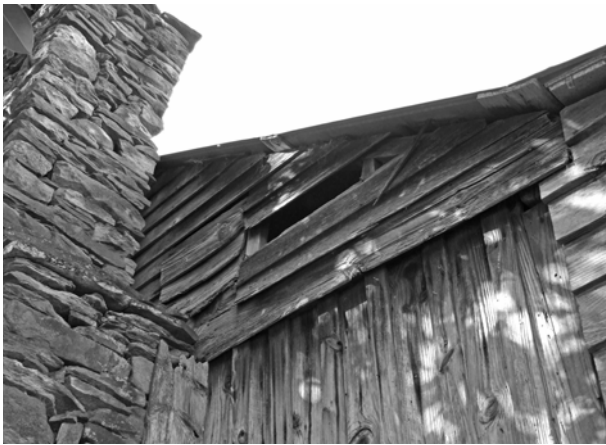
FIGURE 94. View of original siding in east gable, assumed to be contemporaneous with that in the west gable.
