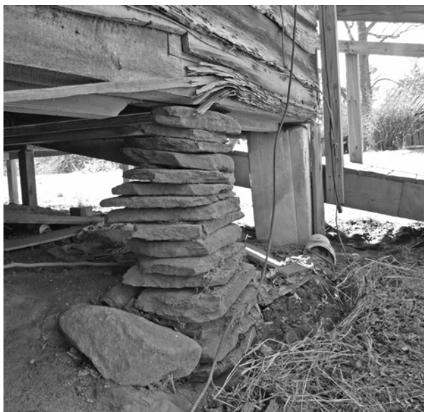
FIGURE 49. View of stone pier at splice in west sill of 1927 addition, with the marble pier at the southwest corner of the addition visible beyond.
