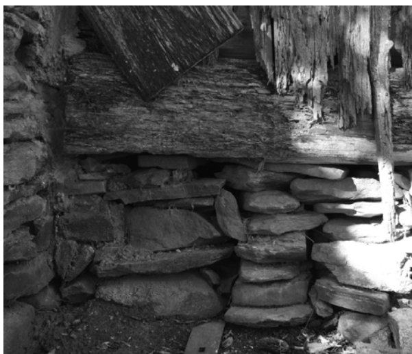
FIGURE 10. View of deterioration at east end of log pen.
