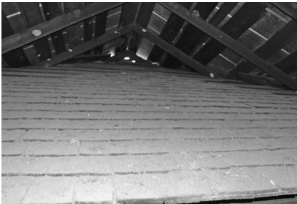
FIGURE 40. View of wood-shingle roofing that survives on what was the rear (south) slope of the roof of the 1925 addition.
