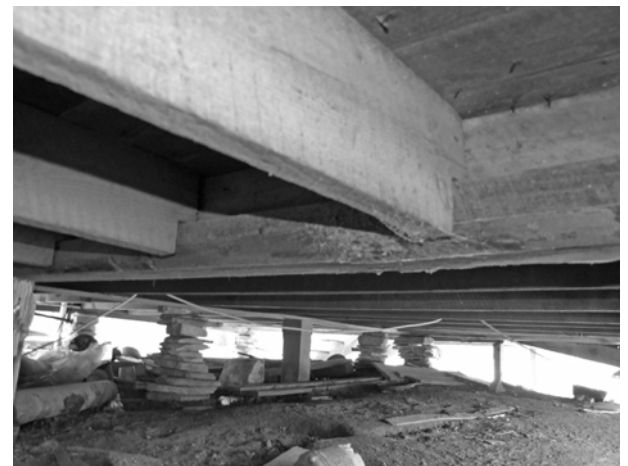
FIGURE 72. View southeast of typical floor joist, ledger, and sill connection in 1925 addition.
