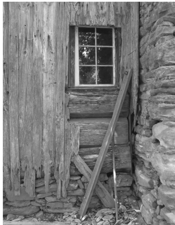
FIGURE 96. View of deteriorated board-and-batten siding at east end of log pen.
