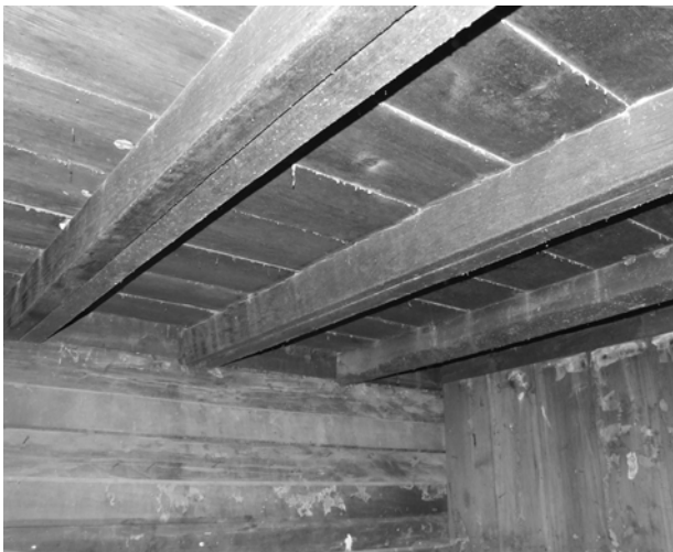
FIGURE 118. View of typical ceiling condition in log pen, southwest corner of Room 101.
