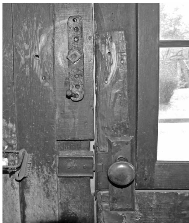
FIGURE 92. View of home-made pivot latch and manufactured rim lock on Door D-4 at rear of 1927 addition.
