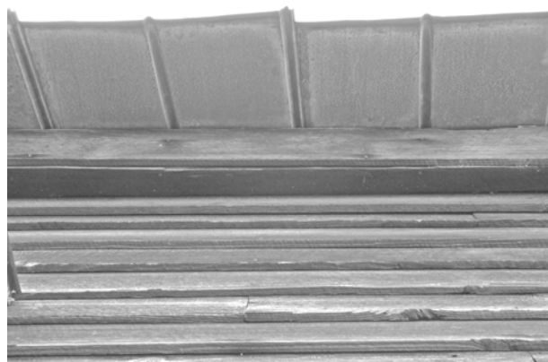
FIGURE 108. View of roofing, soffit, and fascia on front of 1925 addition.
