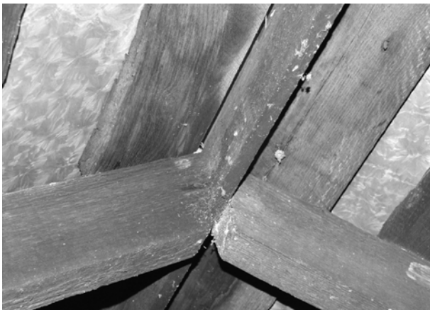
FIGURE 68. View of typical ridge rafter connection in log pen.
