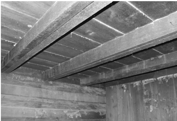
FIGURE 67. View southwest of typical floor joists for loft floor of log pen.
