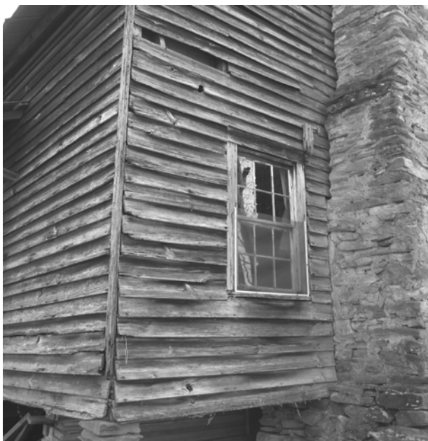
FIGURE 97. View of deteriorated siding and trim at northwest corner of 1925 addition.
