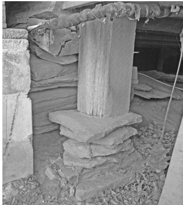
FIGURE 48. View of piers at junction of northwest corner of log pen and the 1925 addition. Left to right, 1998 CMU pier; center, 1840s stacked-stone pier; right 1925 stone pier with wood post.
