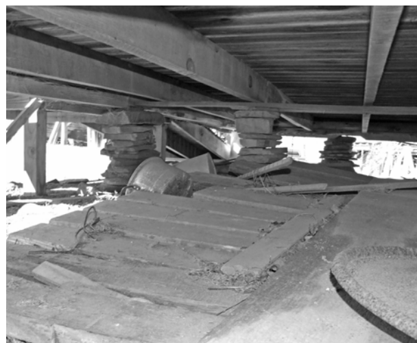
FIGURE 50. View west-southwest under 1927 addition showing pier at center of south sill, left of center, and a second stone pier to its left supporting the end of the “shake sill” running perpendicular to the joists.
