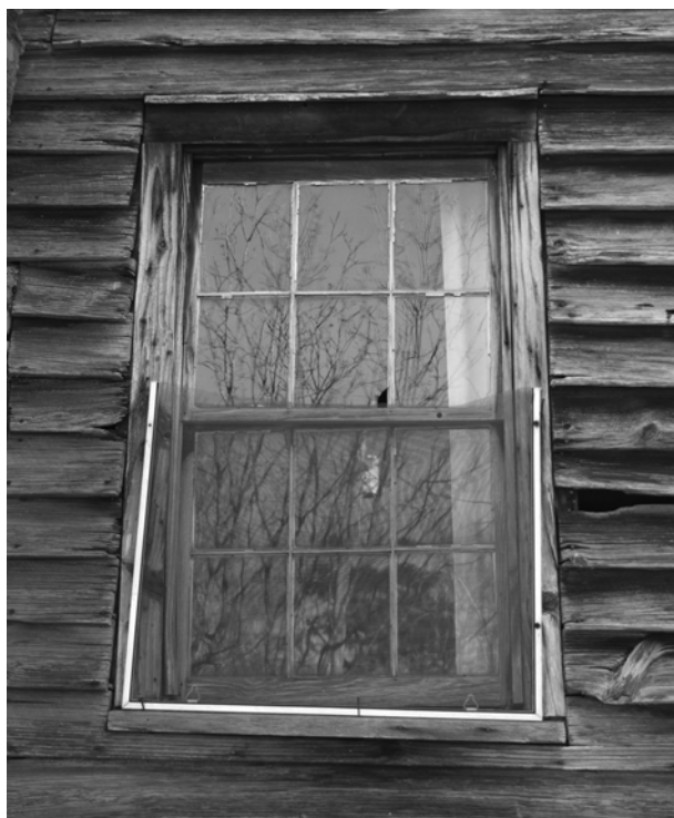
FIGURE 19. View of typical six-over-six, single-hung window in 1920s additions.
