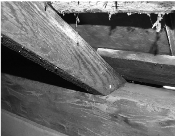
FIGURE 70. View of typical rafter connection to top plate of log pen.
