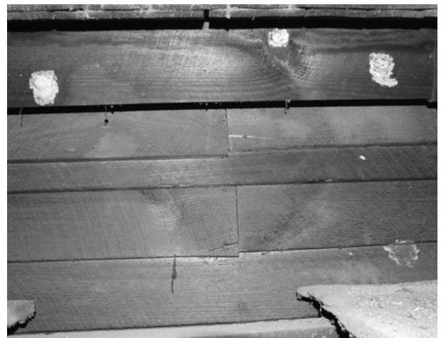
FIGURE 38. View of siding that remains intact and un-eroded on the south side of the 1925 addition, visible above the kitchen ceiling.
